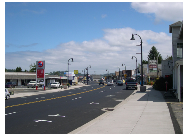
Waldport, after under-grounding utilities
