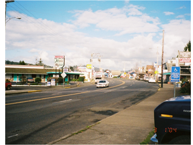
Waldport, with utilities
