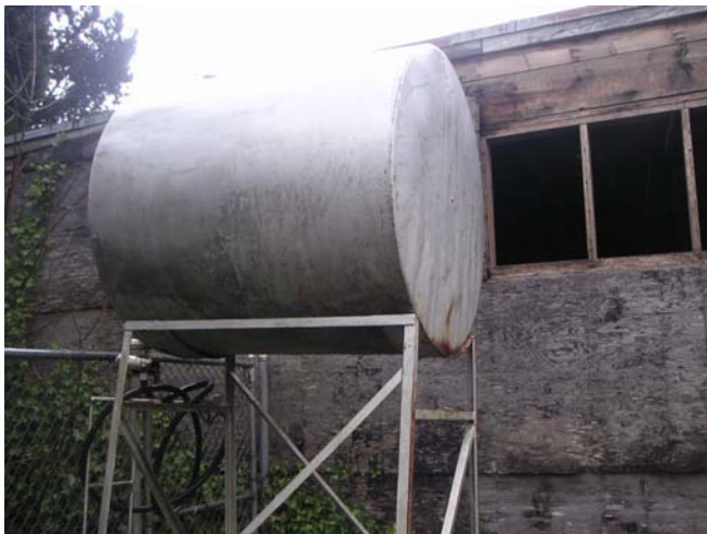
Photo 11: AST located South of Bus Barn
