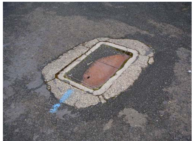
Photo 6: Presumed Fill Port for UST in Middle School Parking Lot
