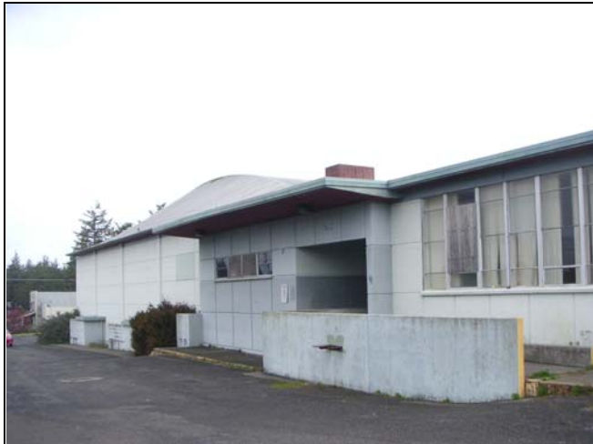
Photo 1: View of West Elevation of Middle School and UST location, Propane Tank in vault against wall
