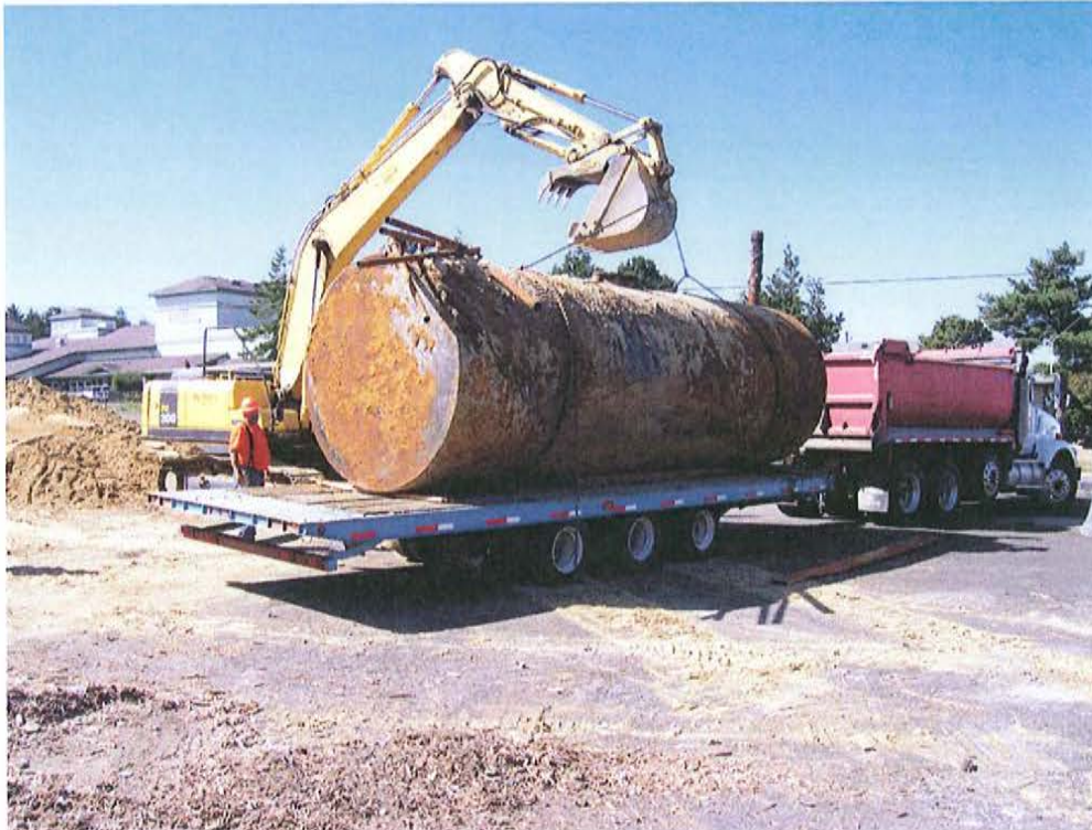
Photo 4: Opposite side of tank.
