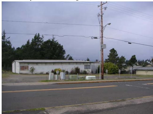
Photo 3: View of Warehouse, View Facing West from Middle School
