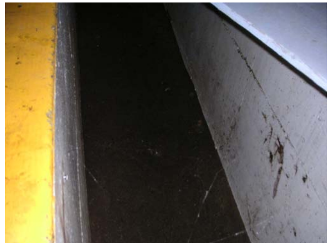
Photo 12: Lube Pit in Maintenance Building
