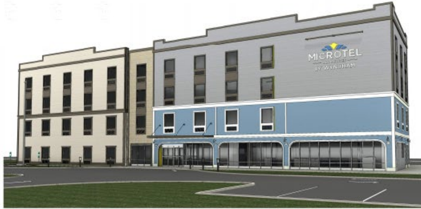
1 VIEW FROM SW CORNER
