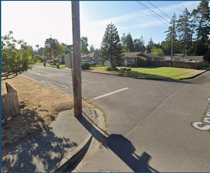
Incomplete Sidewalk Networks
