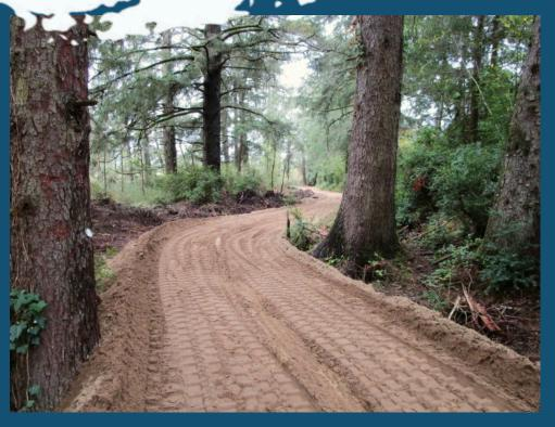
Laskey-Clifton has continued to work on the trailhead on Redwood Street and estabilished the path along the estuary. This includes slope stabilization, stormwater lines, geothermal fabric, mulched material, crushed rock, and more.
