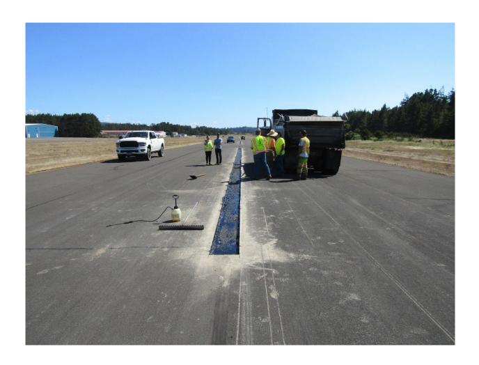
Wednesday, the contractor slurry sealed the runway, taxiway and taxi lanes. A slurry seal is a homogenous mixture of emulsified asphalt, water, well-graded fine aggregate (for our project a fine sand material) and mineral filler that has a creamy fluid-like appearance when applied. Slurry seals are used to fill existing minor pavement surface defects, improve skid resistance and provide additional life to the existing pavement.
