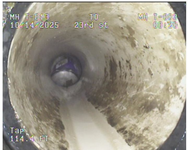
Clean Sewer Pipe
