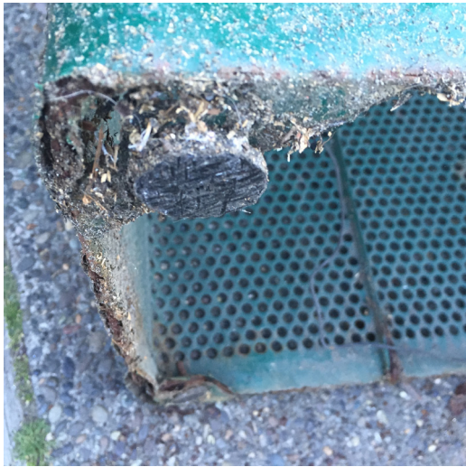
Trash Bins Need to be replaced
