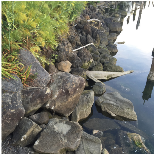
Near Water, Tide work?
