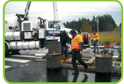
BayFilter System Cleanout
