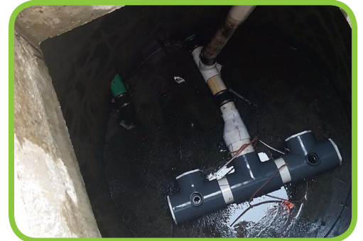
Manifold Tee View of a Cleaned System
