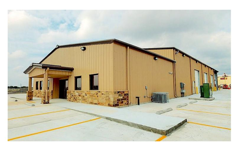
The building pictured above exhibits a mostly average metal building appearance with a fairly flat roof slope and walls nearly flush to the roofline.
