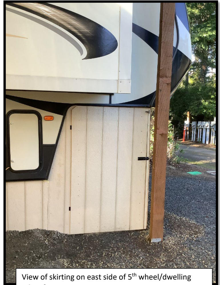
This image is intended to show a door to access under the skirting and that the skirting does to open at the front to allow the vehicle to be easily towed or removed from the lot.
