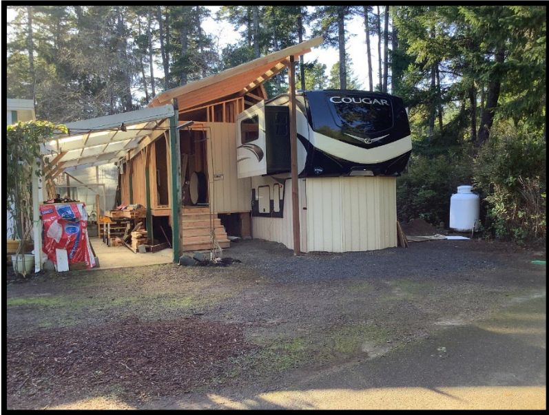
86 Outer Drive: View from Outer Drive facing south. • New propane tank (permits pulled and issued) visible right on east side of the property. • 5 th wheel/dwelling and new covered deck with stairs middle • Pre-existing carport structure left
