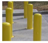
base or foundation. Safety will be enhanced if the bollards have reflective tape or some type of illumination (MUTCD; Bike Blogs). Any feature used in combination with the bollards, such as a fence, must not create a hazard to occupants of any vehicle or anyone in the dining area during a crash or during any time. Materials should not be used that can break apart and potentially become projectiles.
