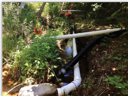
Figure 4-36 - Private drainage piping discharging into ditch. Efforts made by Seabrook Townhomes residents to alleviate flooding
