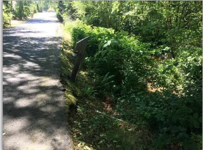
Figure 6-28 - Eroded edge of pavement. Address by replacing/extending culvert and adding fill material
