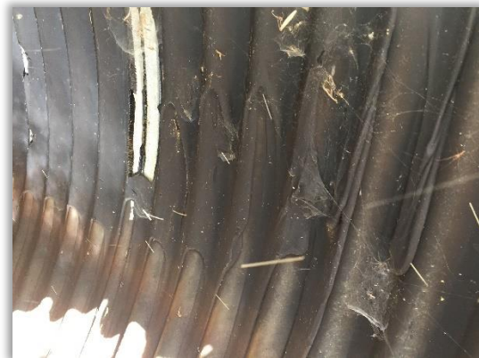
Figure 5-11 - Coal-tar epoxy present on pipe wall
