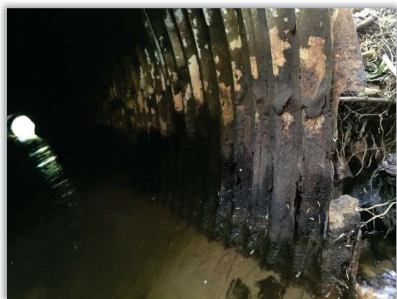
Figure 5-2 – Deteriorated factory coating
