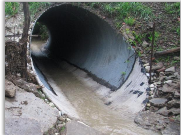
Figure 6-27 - Geosynthetic cementitious composite mat applied to CMP culvert to extend lifetime of culvert (example)
