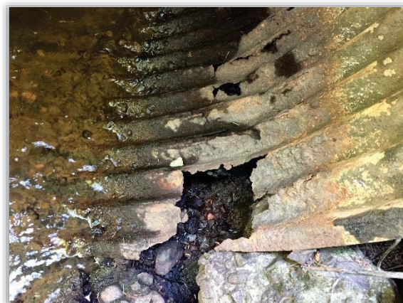
Figure 5-3 - Evidence of severe corrosion in pipe wall
