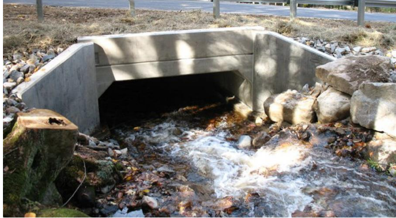
Figure 6-24 - Photograph of open bottom concrete box culvert.
