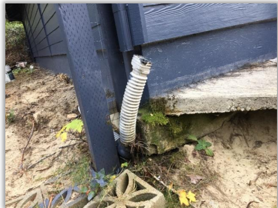
Figure 6-8 - 3515 Rhododendron Drive 3-car garage foundation exposed
