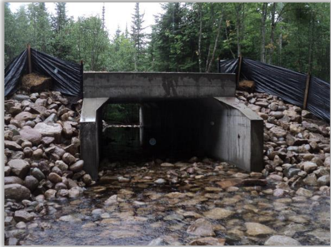
Figure 6-25 – Example of open bottom box culvert. Potential future solution @ 23 rd St crossing
