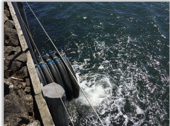
Figure 5-19 - 36-inch outfall constructed of ADS
