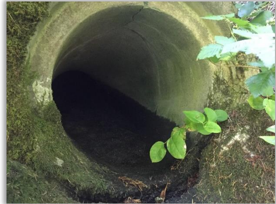
Figure 5-6 - Outfall pipe is sloped uphill in the direction of flow, causing sedimentation
