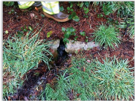
Figure 4-20 - Intentional break in 10" transite pipe for drainage
