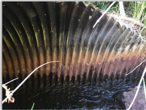
Figure 6-26 - Evidence of corrosion in existing pipe wall
