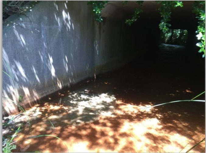
Figure 5-17 - 10' x 8' box culvert crossing Rhododendron Drive
