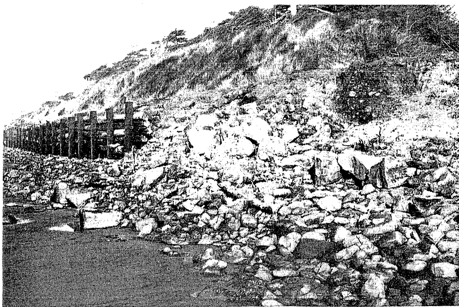
Figure 33. The wood piling bulkhead built on Netarts Spit to stop wave attack of the dunes.
