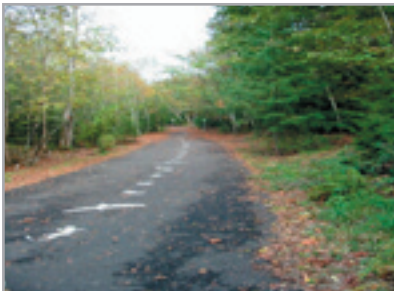
Oaks Bottom Connector - existing dirt road was paved, some slopes greater than 5%
