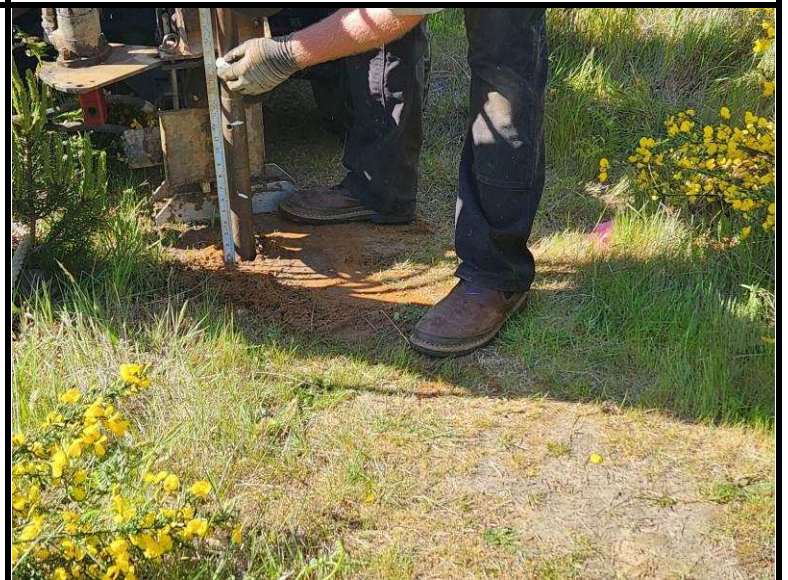
Drilling of boring B-6
