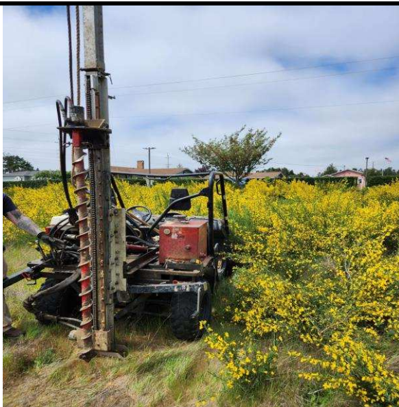
ATV mounted drill rig used for borings
