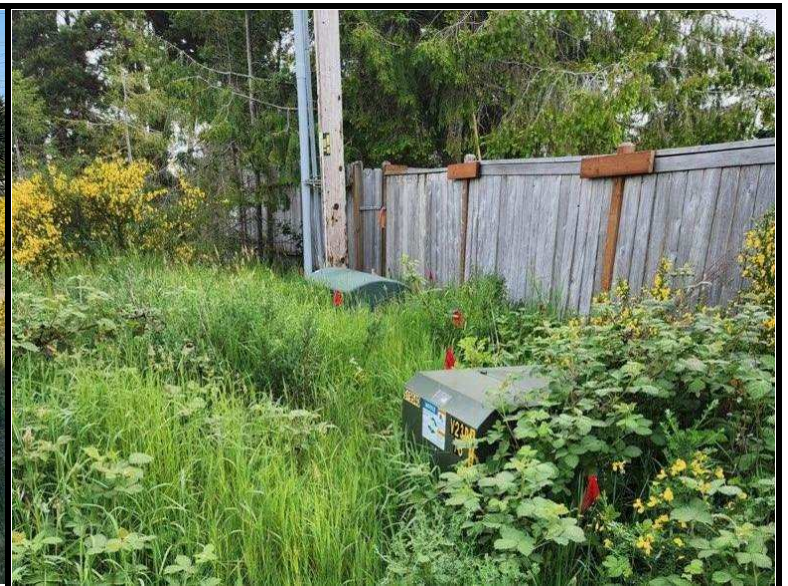
Utilities located near northeast corner
