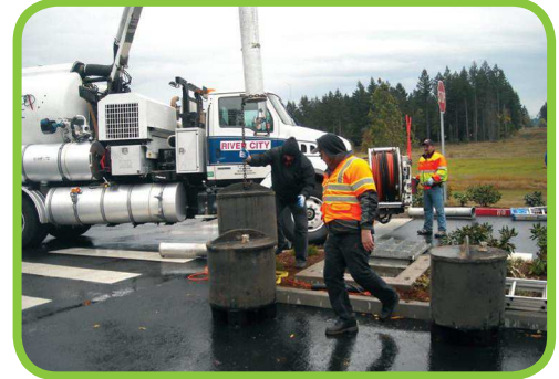
BayFilter System Cleanout
