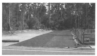
small dog areas: excavated for the stormwater quality swale: installed/placed the three part blend (soil mix: 1 part compost, part native sand, and one part sandy loam) for the
