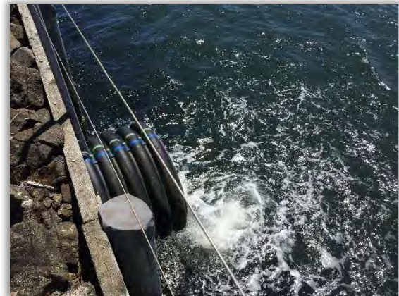
Figure 5-19 - 36-inch outfall constructed of ADS
