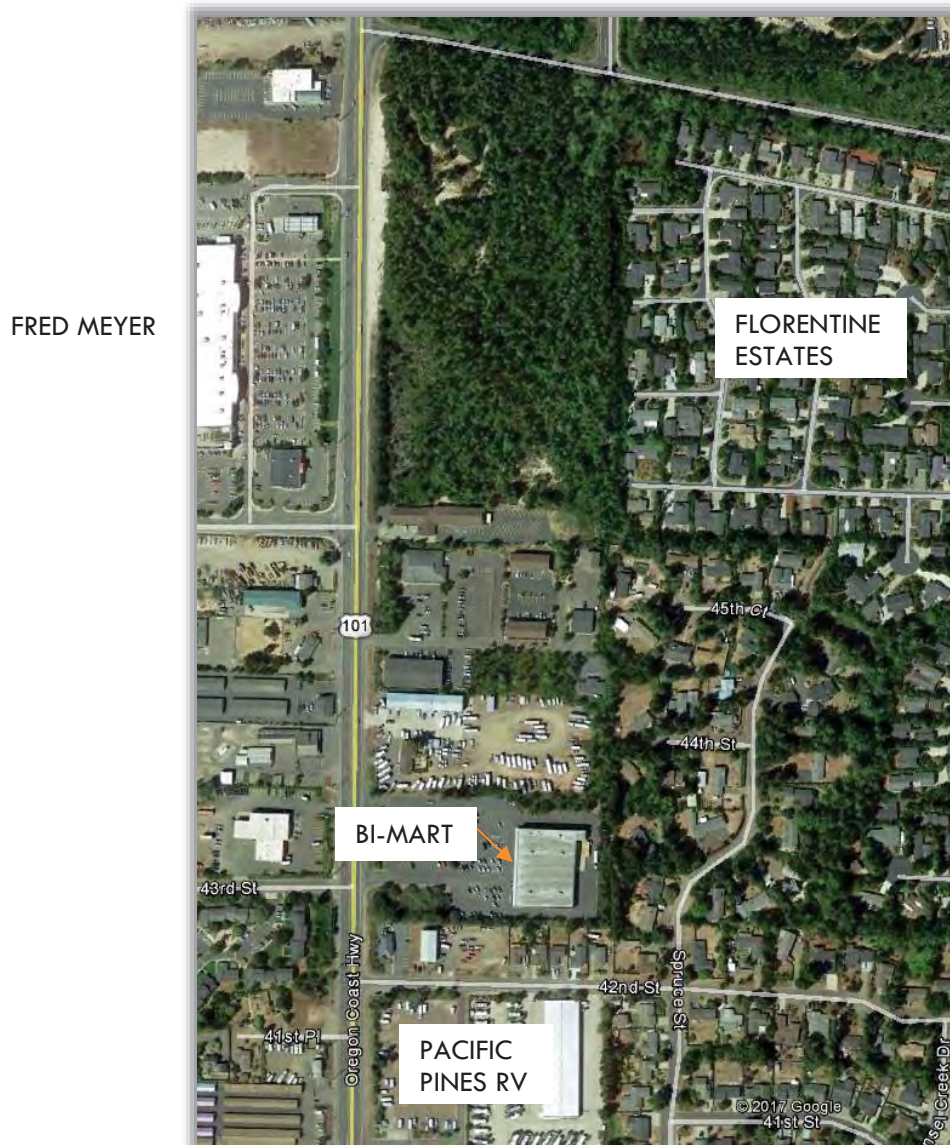
Figure 4-3. Aerial Map of Stormwater Tributary Area
