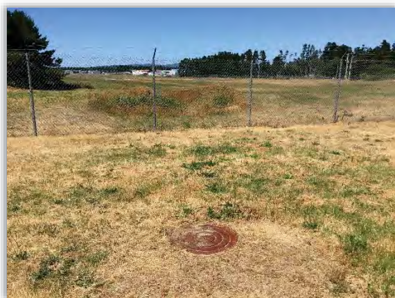
Figure 4-31 - Airport drainage ditch & manhole @ 12th Street R-O-W, SW end of airport property
