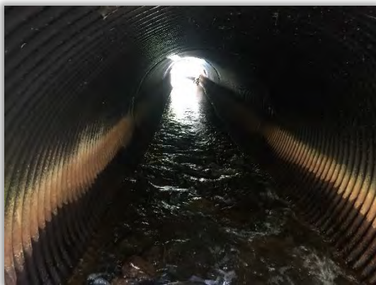
Figure 5-10 - Inside of 72-inch culvert, level of water stains suggests sufficient capacity
