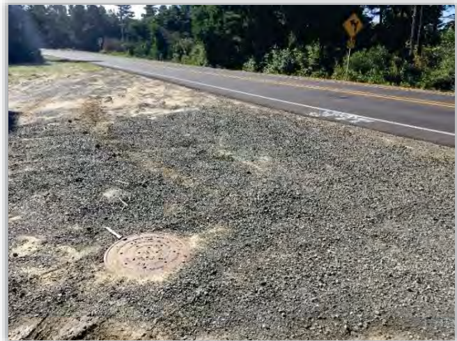
Figure 4-19 – Flow control manhole w/ no outfall constructed yet
