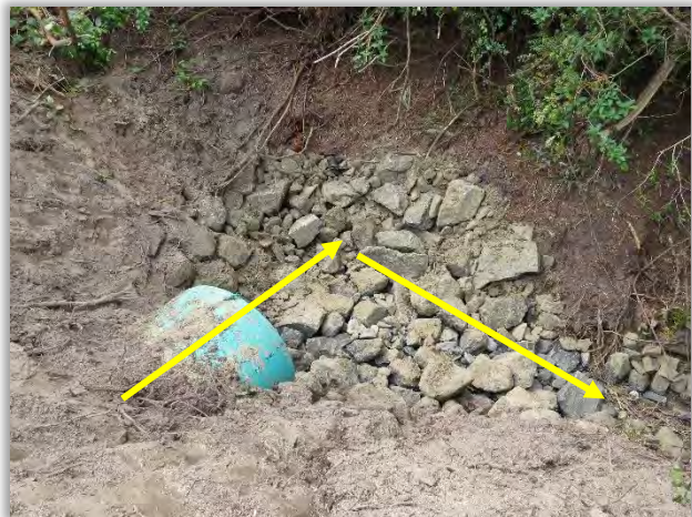
Figure 6-12 - Inlet into Bud's Ravine (90-deg angle turn)
