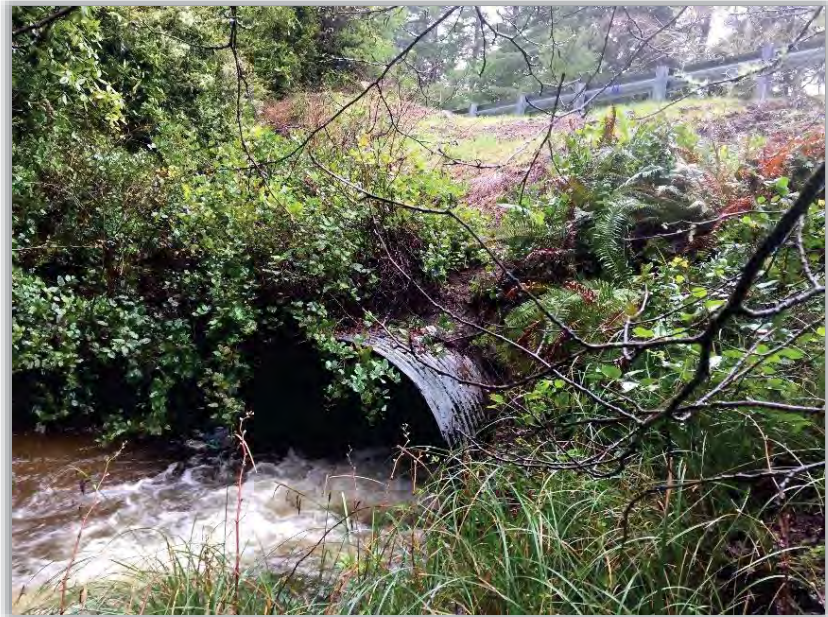
Figure 5-1 - 84-inch CMP culvert, outlet side, looking NE
