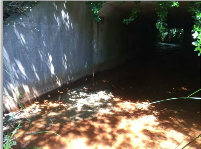
Figure 5-17 - 10' x 8' box culvert crossing Rhododendron Drive
