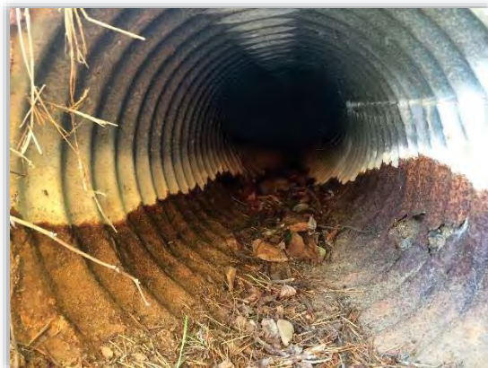
Figure 4-44 - 18-inch CMP culvert at top of bluffs on North Jetty Road
