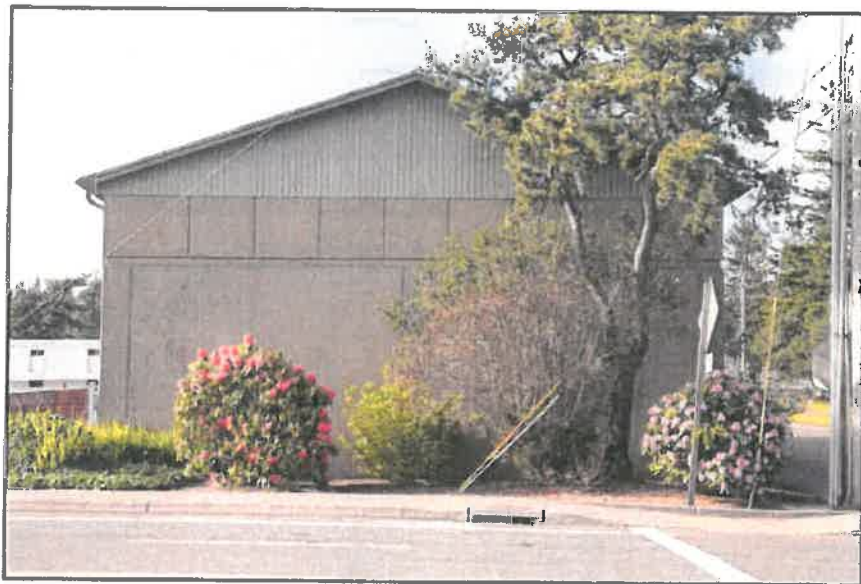
South Facing Wall, 37 ft x 15.5 ft
