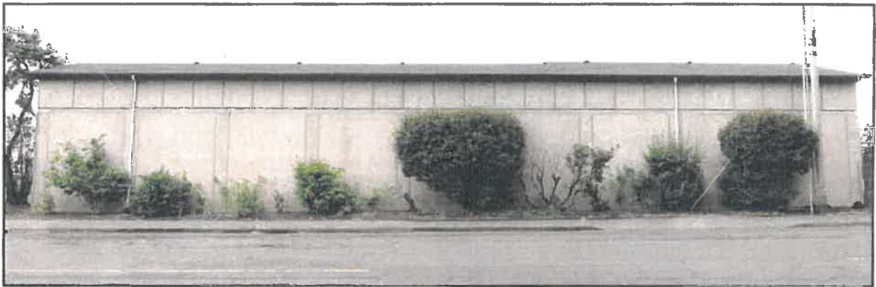
East Facing Wall, 108 ft x 15.5 ft
