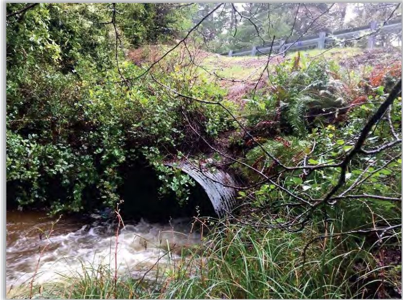
Figure 5-1 - 84-inch CMP culvert, outlet side, looking NE
