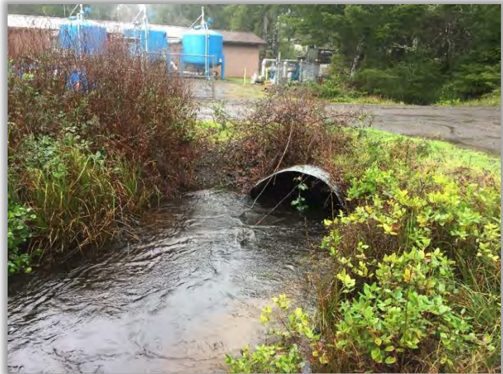
Figure 5-14 - 60-inch CMP culvert at WTP
