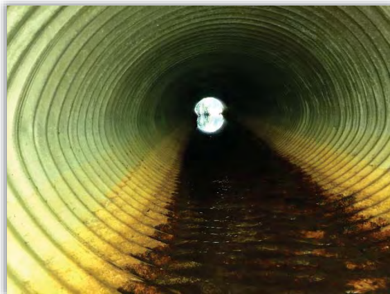
Figure 4-10 - 36" CMP culvert at Munsel Lake Rd.
