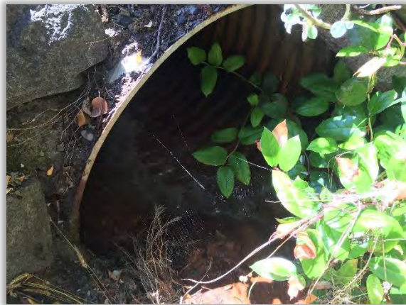
Figure 5-18 - 36-inch CMP pipe from box culvert to river
