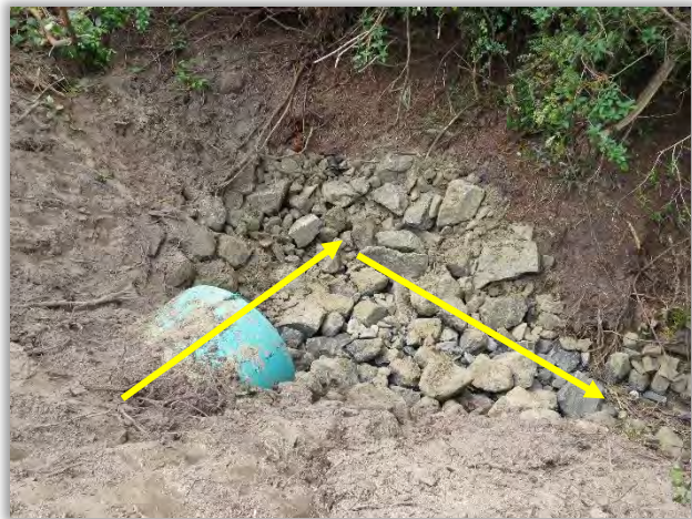
Figure 6-12 - Inlet into Bud's Ravine (90-deg angle turn)
