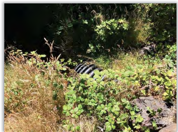
Figure 4-32 - 36" ADS culvert outlet for drainage under 12th Street right-of-way
