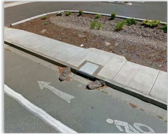
Figure 4-27 - Biorolls placed by curb inlet
