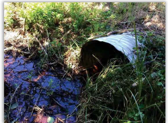
Figure 4-11 - 36" CMP Culvert at Munsel Lake Rd.
