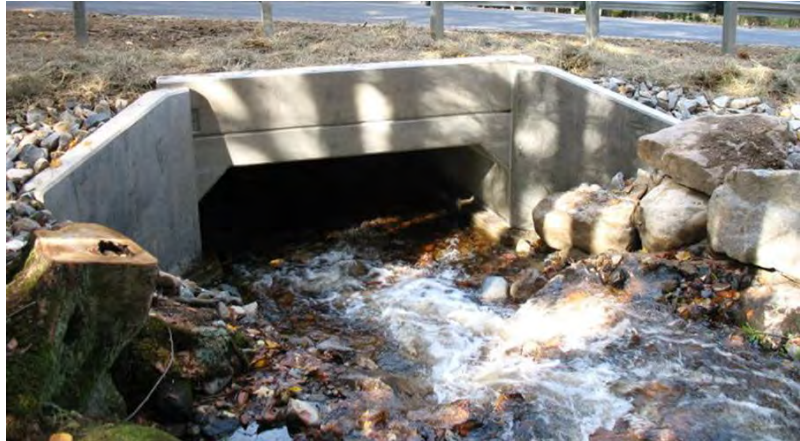
Figure 6-24 - Photograph of open bottom concrete box culvert.
