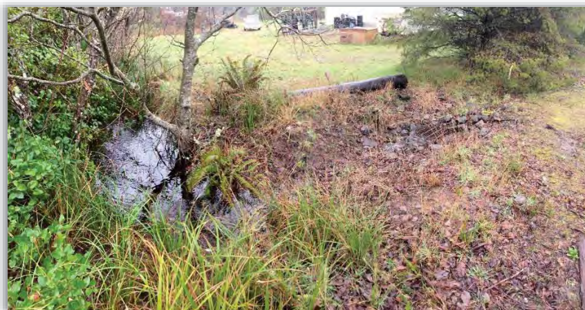
Figure 4-7 - Siefert Ditch with Catch Basin
