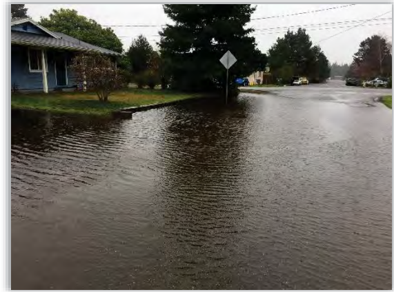
Figure 4-2 - Spruce Street, looking SE
