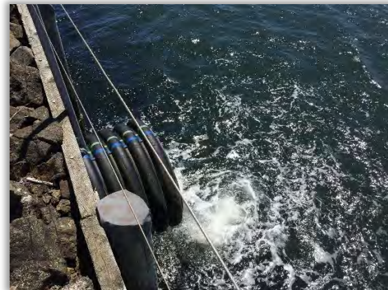
Figure 5-19 - 36-inch outfall constructed of ADS
