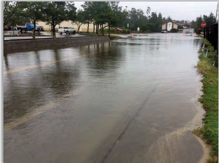
Figure 4-4 - 46th Street, looking East
