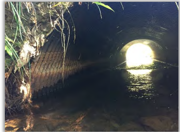
Figure 5-16 - Inside of WTP culvert
