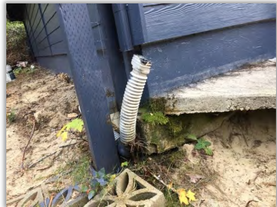
Figure 6-8 - 3515 Rhododendron Drive 3-car garage foundation exposed
