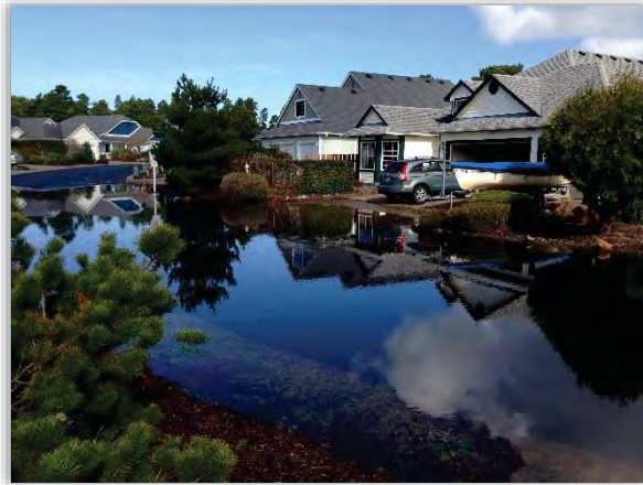
Figure 4-15 - Spyglass Lane flooded after water surcharged out of catch basins
