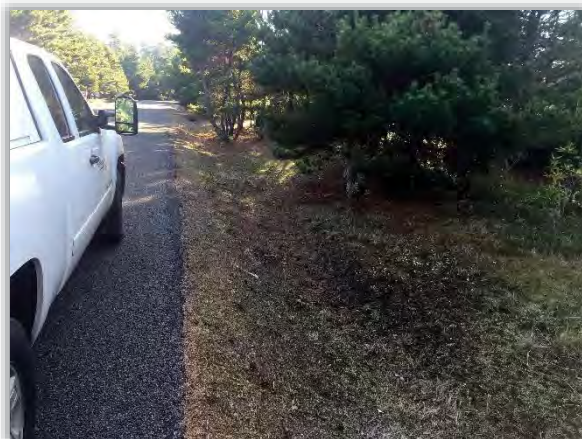
Figure 4-41 - Roadside Ditch (Sandrift Street)
