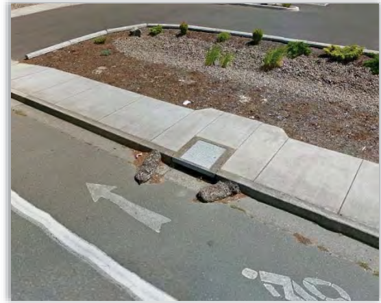
Figure 4-27 - Biorolls placed by curb inlet
