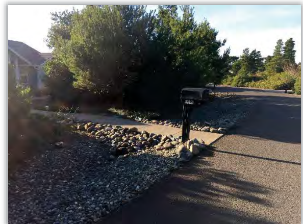
Figure 4-42 - Roadside infiltration swale (Saltaire Street)
