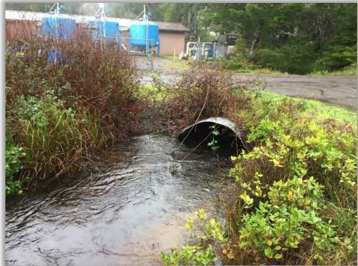
Figure 5-14 - 60-inch CMP culvert at WTP
