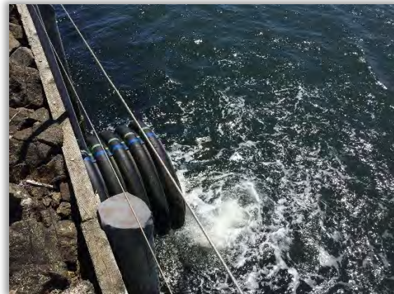
Figure 5-19 - 36-inch outfall constructed of ADS
