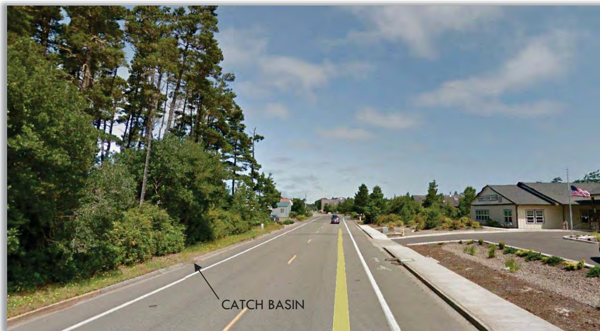
Figure 4-26 - Kingwood Street at Florence Senior Center, looking North
