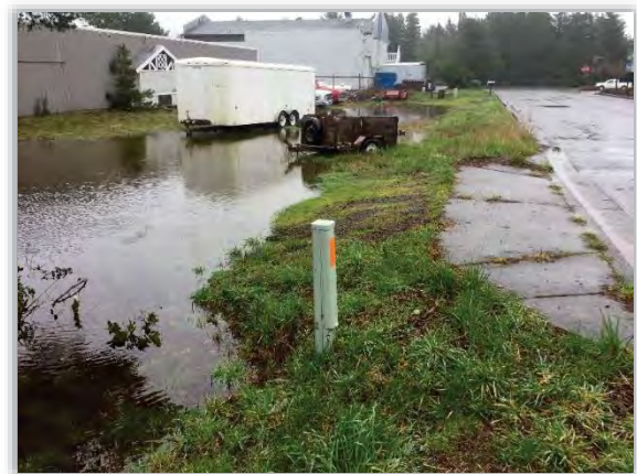
Figure 4-22 - North side of 28th Street, looking east from Pine Street
