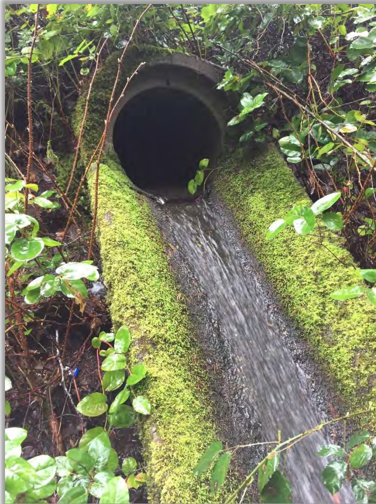
Figure 5-7 - Concrete chute channeling flow down into Munsel Creek
