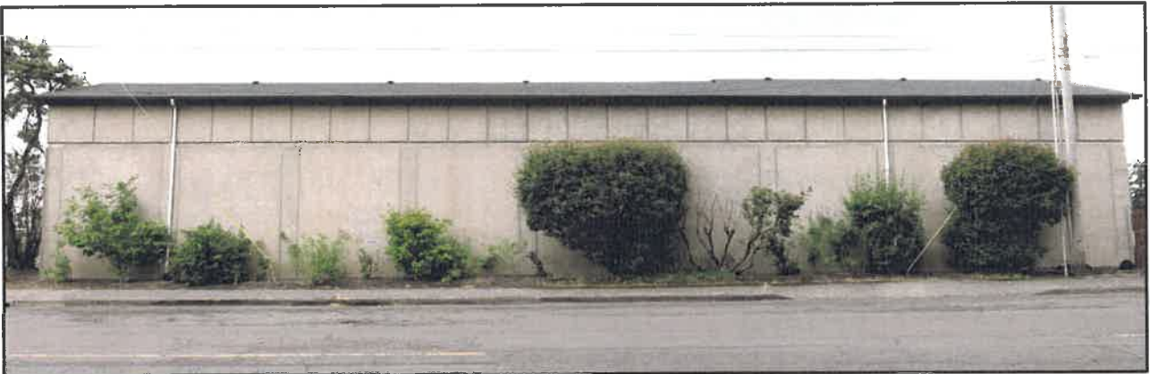
East Facing Wall, 108 ft x 15.5 ft
