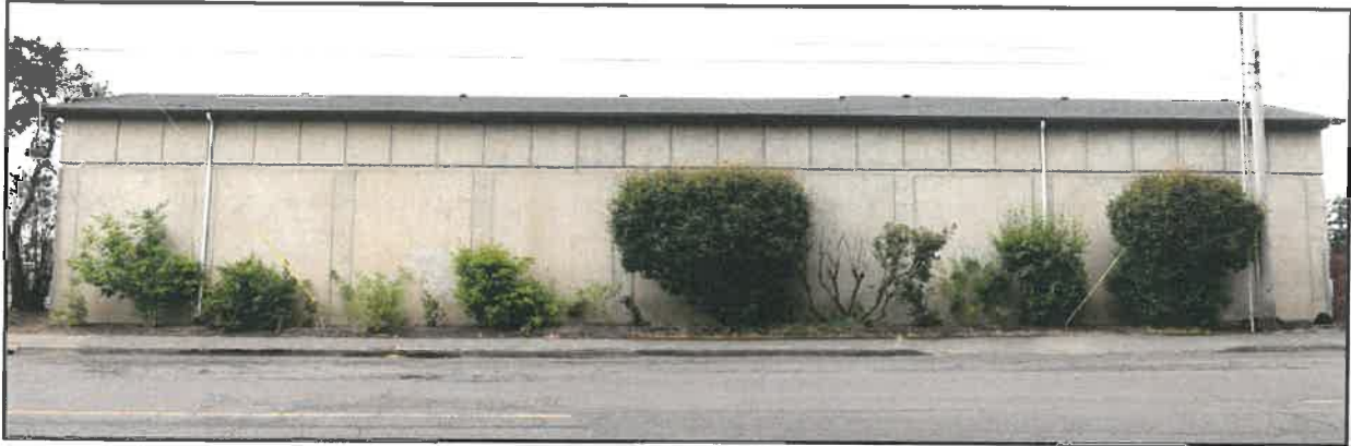
East Facing Wall, 108 ft x 15.5 ft
