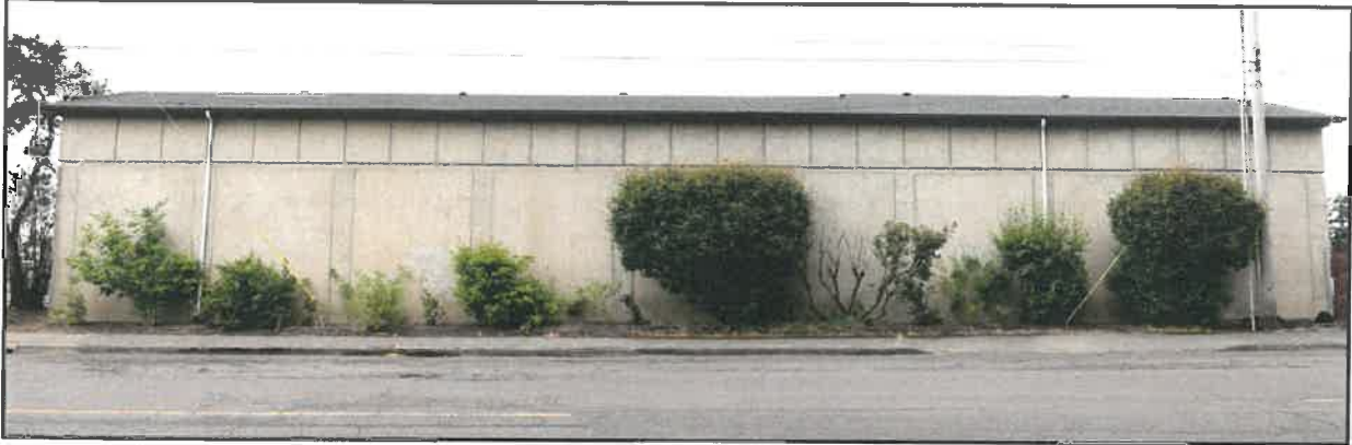
East Facing Wall, 108 ft x 15.5 ft
