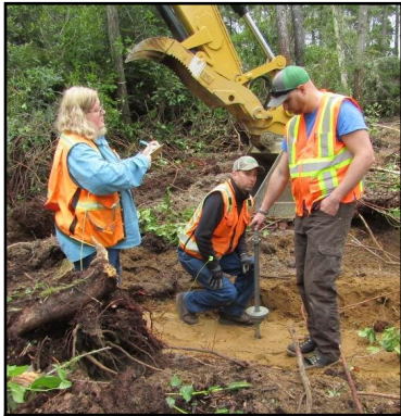
Crews collecting soil samples at the new Public Works Facility site.
