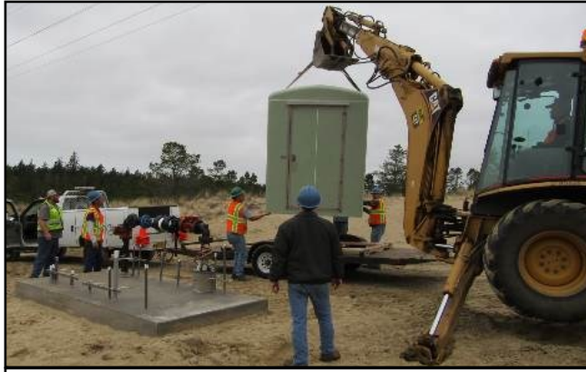
Crews set the new well enclosure for Well #3A.
