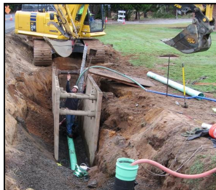
New sewer main installed along Munsel Lake Road.
