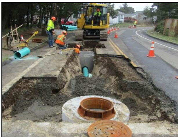
Crews installing new stormwater system on 35th Street.
