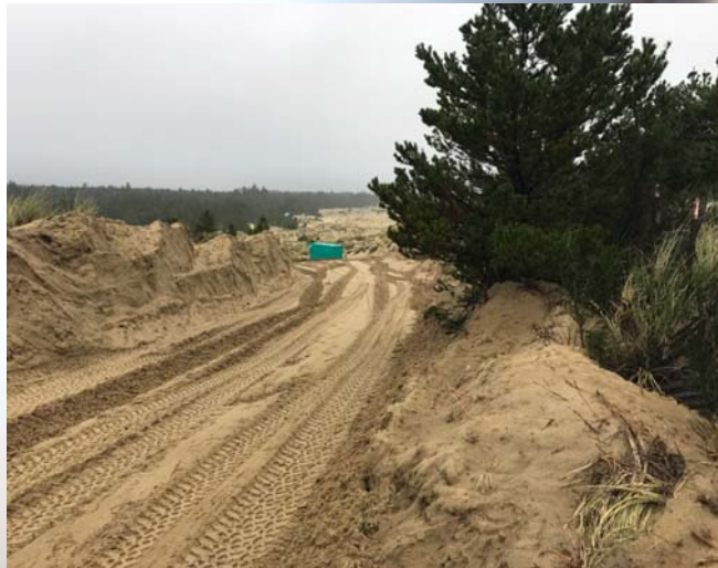
Sand is cut and pushed to create a path to Well #8
