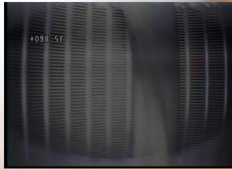
Image of well screen after cleaning/rehabilitation
