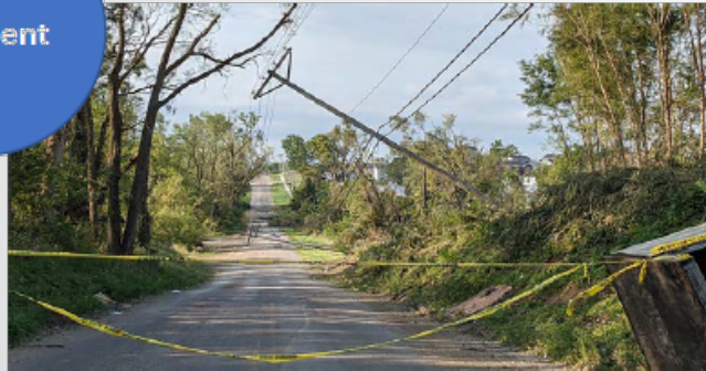
Straight-line wind damage | via AP Images
