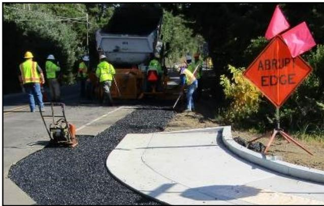
*The base lift of permeable paving being installed for the Rhododendron Drive shoulder extension.*
