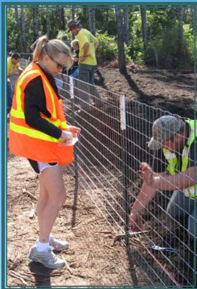
City Manager Jacque Betz (left) and Public Works crew member Sean Selig work on a fence at the new Singing Pines Dog Park on Make-A-Difference Day, July 21st. Hundreds of volunteers came together that sunny Saturday to work on the parks, clean beaches and fundraise.
