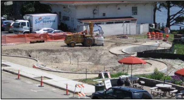
Tom Ayres General Contractor continues construction on the Siuslaw Interpretive Center.
