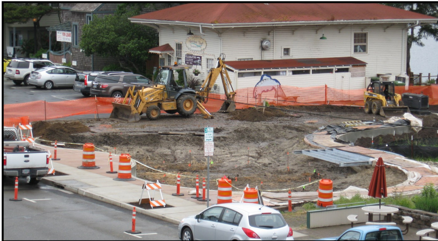
Siuslaw River Bridge Interpretive Center under construction on May 29, 2013.
