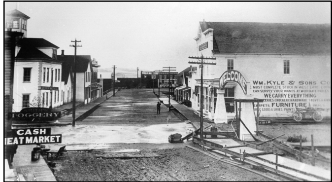
Planked street and sidewalks at the west end of Front Street with the first attempts at paving shown near the center of the photo.
