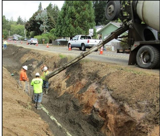
Placing CLSM (controlled low-strength material) over the new sewer line. CLSM is a self-consolidating, cementing material used as backfill as an alternative to compacted fill.
