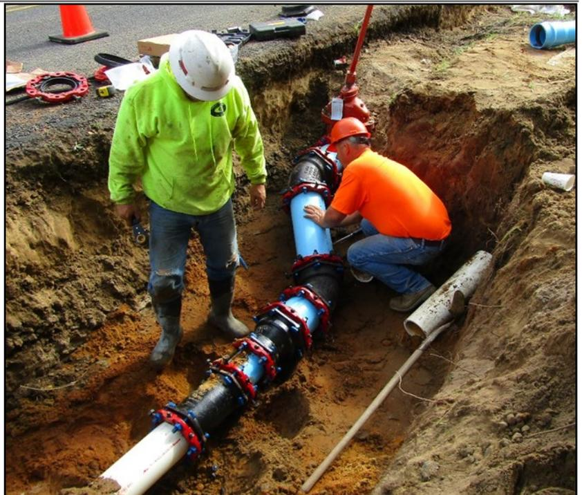
Crews from Morello Construction preparing the final tie over from the existing 6-inch water system (white pipe) to the new 8-inch (blue pipe) water system.
