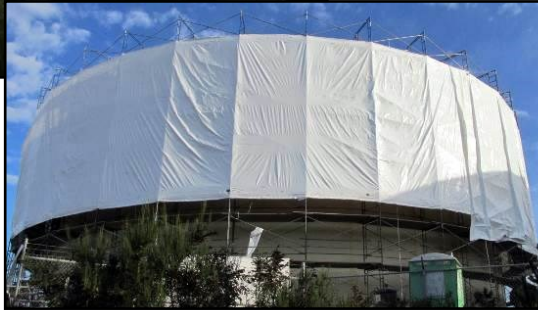
Above: Crews install the scaffolding around the west water tank.
