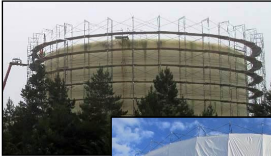
Above: Crews install the scaffolding around the west water tank.
