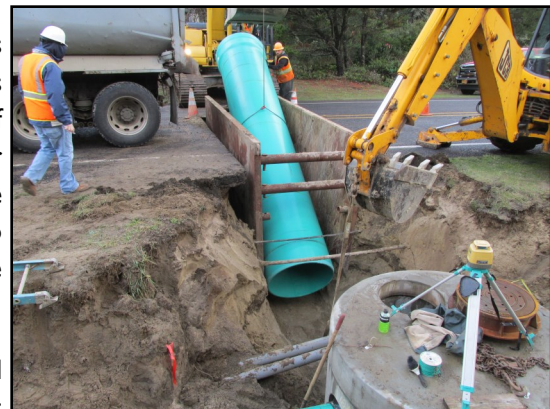
Contractor installing a section of 42-inch stormwater line across Rhododendron Drive.
