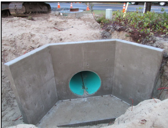
New inlet structure for the 42-inch stormwater system.
