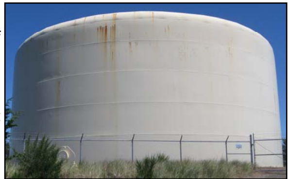
The west reservoir near Sandpines Golf Links. Notice the paint system failure and rust developing on the tank.
