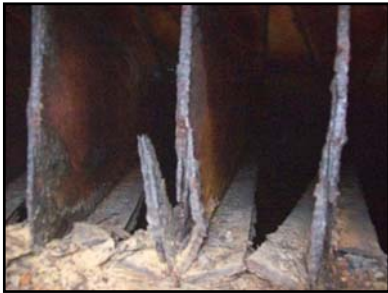
Roof support beams for the 500,000 gallon tank at Rhodoview Dunes.
