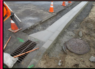
New Curbs and Gutters
