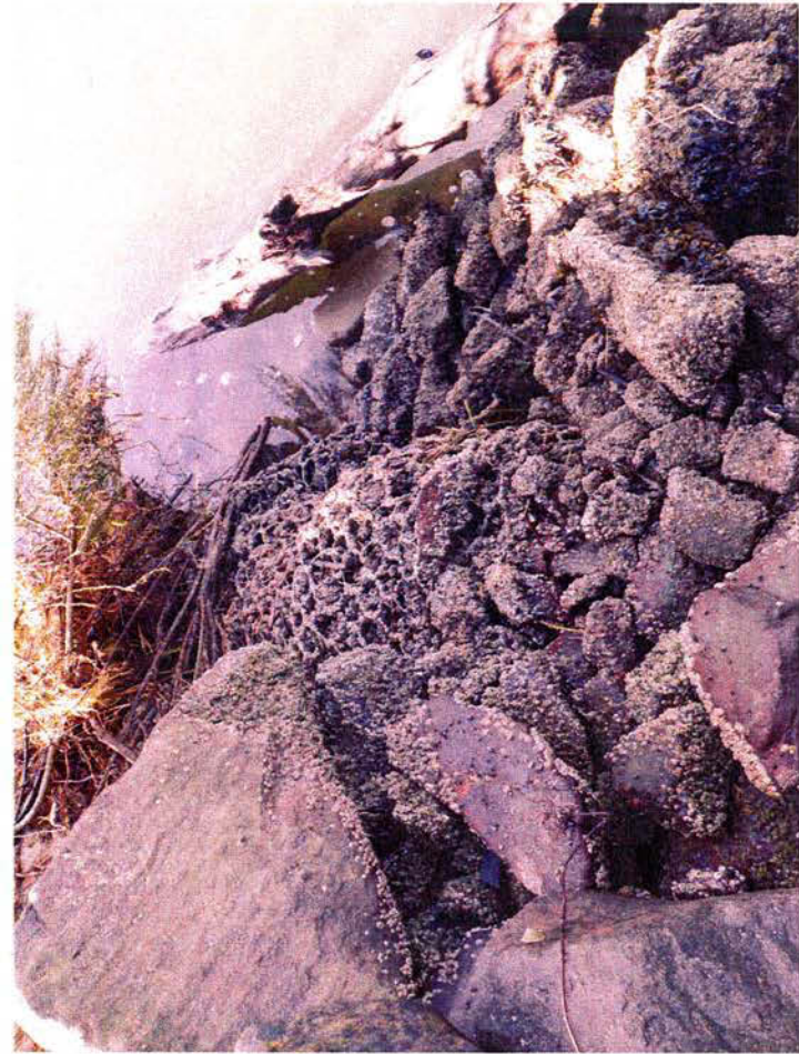
Gabions involved in failure at N end of slope movement deposit. Baskets have been deflected westward by the movement.
