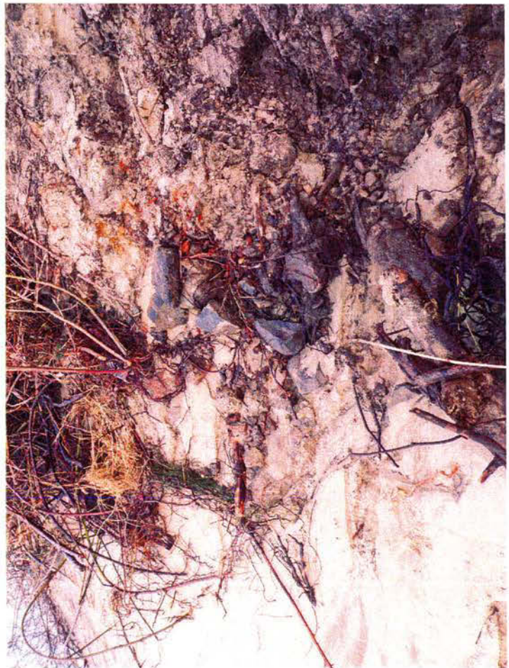
Rip rap exposed in S central portion of the toe of the slope movement. Sand to left is slope movement deposit in area under water at OHW.
