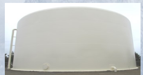
Finished tank with its bright and shiny new coating system.
