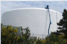
Primer coat applied to tank.
