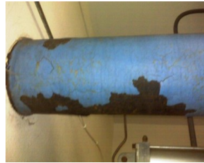
The photo to the left is of a section of pipe at the water treatment plant where the paint coating has failed due to
